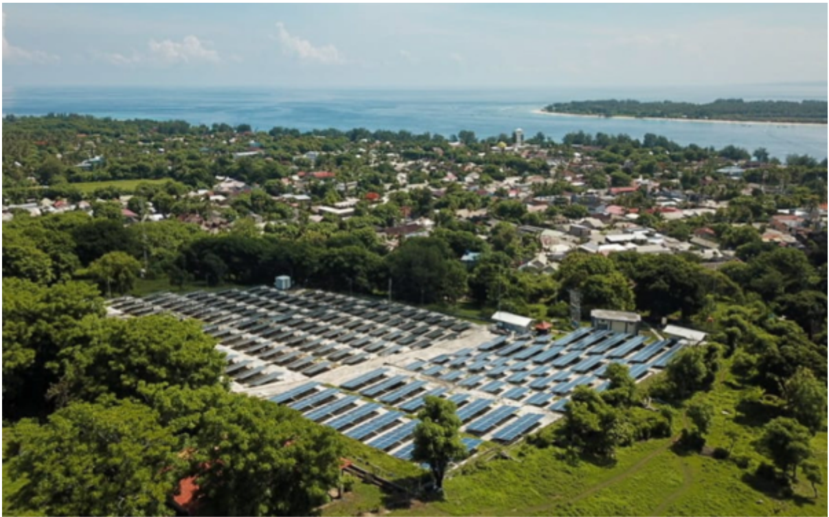
A 600-kilowatt-peak (kWp) solar power plant on Gili Trawangan island in Lombok, West Nusa Tenggara
