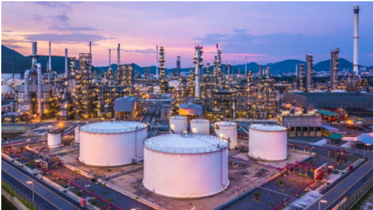
PTT Thailand, Petroleum Factory
